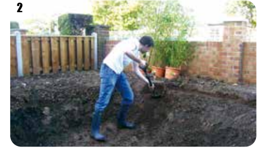
2 Finishing the dig by hand - digging out shelves and smoothing the surface. Get rid of as many stones as you can.
