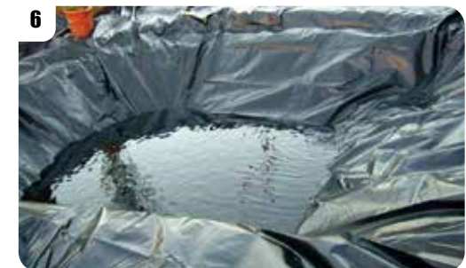
6 Weigh liner edges down then smooth away folds as water starts to fill the pond.
